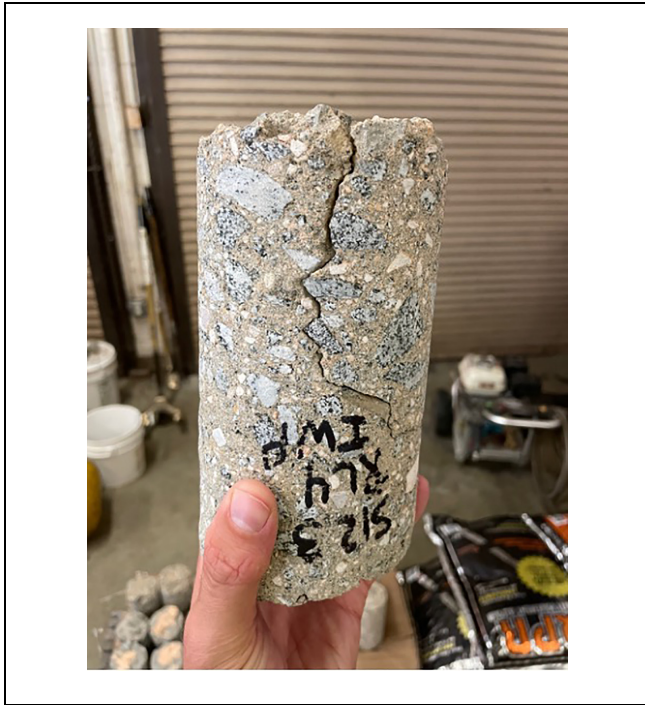
Figure 9. A stabilized base core with a full-depth crack.
